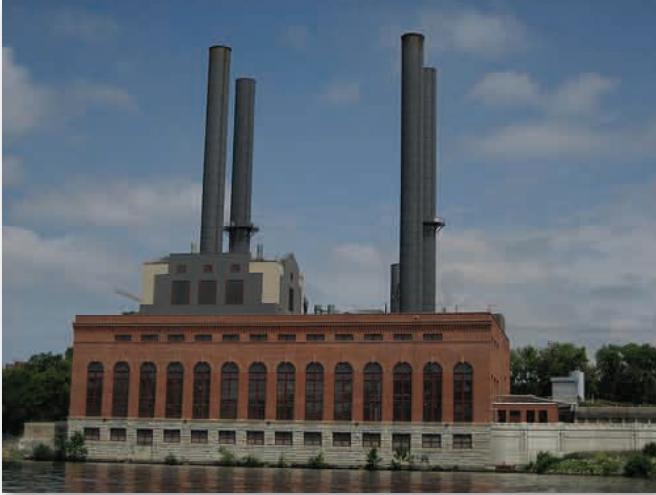
Southeast Steam Plant, University of Minn. campus
