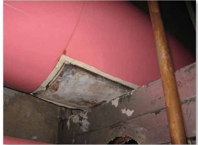
Jacket notched around support, due to space limitations and interferences
