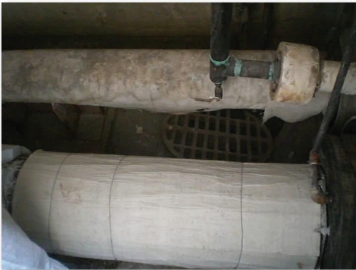
Pyrogel aerogel insulation on pipe
