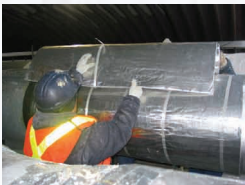
Cryogel® Z insulation rolls delivered, cut to size, and installed.
